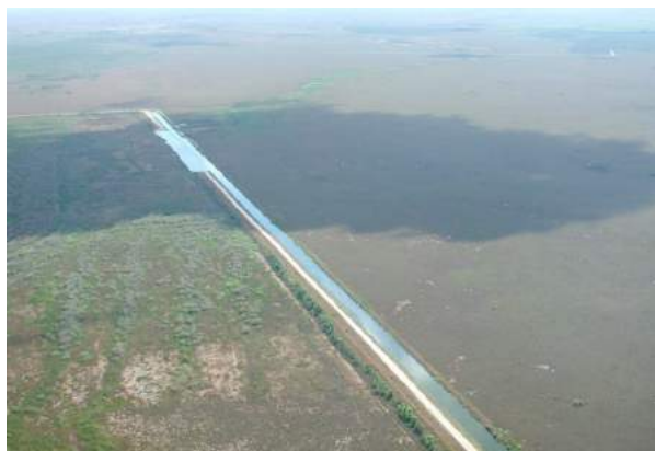
Figure 4.26: Example of levee in the Frog Pond Area (where Site 2 is located). North to south photo of S332 and levee removal on eastern boundary of levee L31 (from FCE-LTER website)
