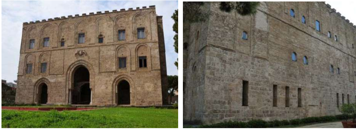
Fig. 4: Big windows for the best captation of sea-wind from East side and smallest windows on West façade, in order to reduce the solar irradiation.
