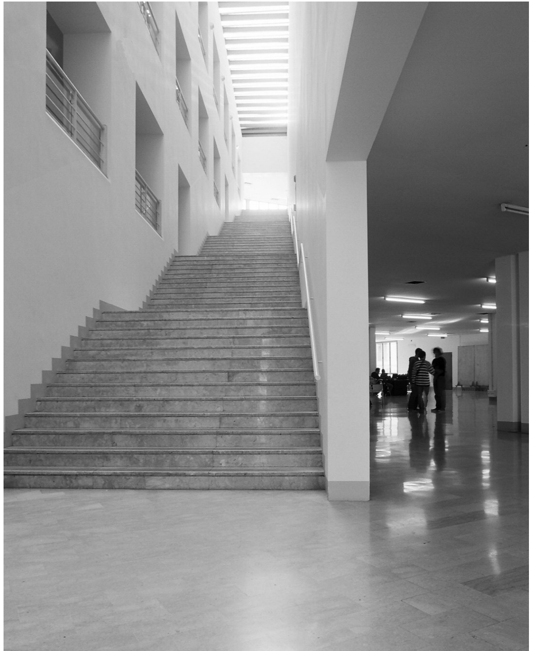
Fig. 7 - The main staircase of the Department of Architecture (photo by S. E. Di Miceli).
