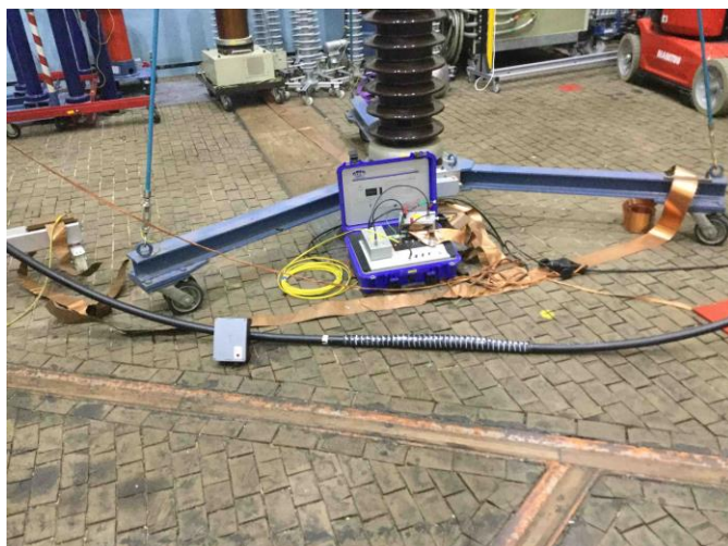
Figure 5-19. Pry-Cam portable placed on left side of the joint
