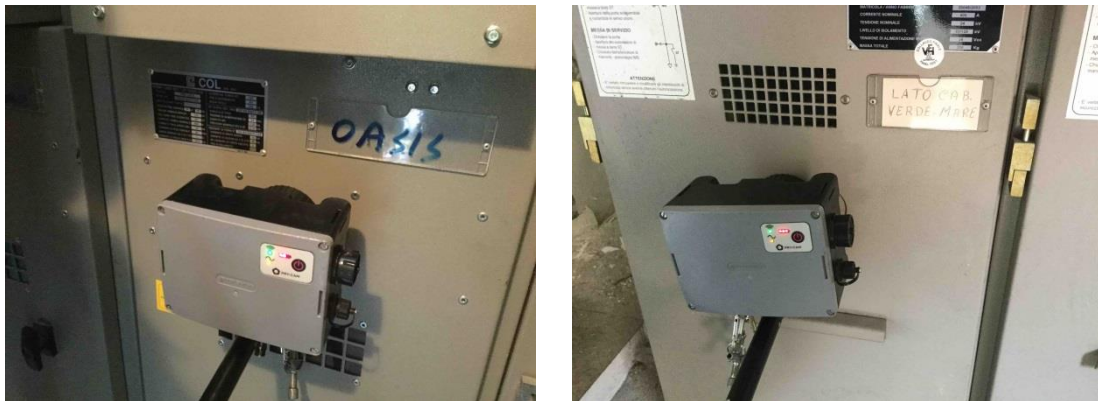
Figure 6-60. Pry-Cam Portable placed on the magazine inspection window
