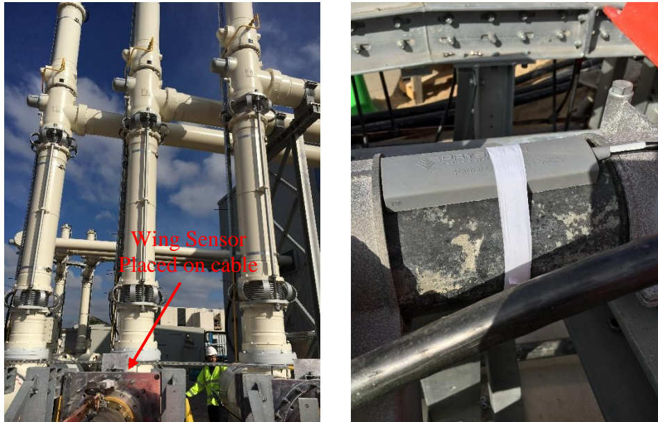
Figure 6-17. Wing Sensor placed on Cable before starting test HV test
