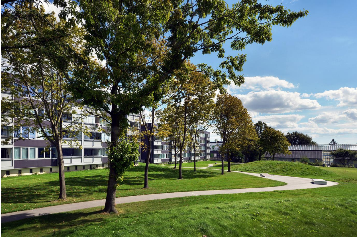
Figure 8.2. Skovgårdsparken after renovation
