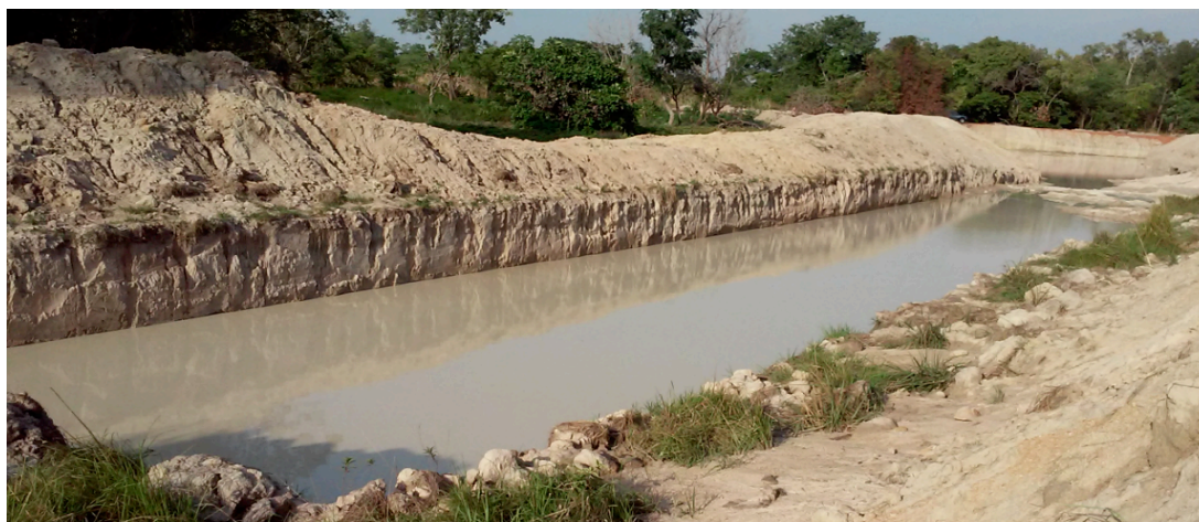
Fig 6: Hydro-agricultural development in progress in the village of Togoniéré
