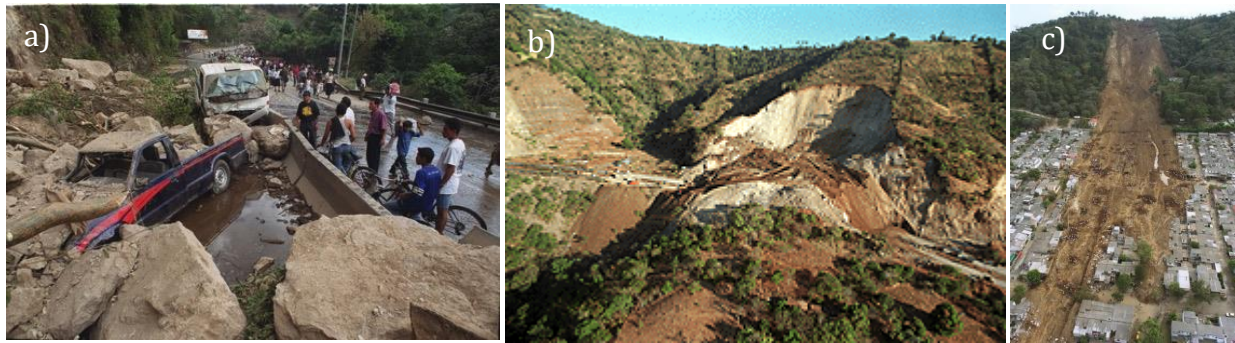
Fig. 4.7 – Landslides triggered by earthquakes in El Salvador January 2001, a) Rockfall in Los Chorros Pan-American Highway (Civil Protection, 2001), b) Curva de La Leona Landslide Pan-American Highway, c) Las Colinas Santa Tecla landslide (Civil Protection, 2001).
