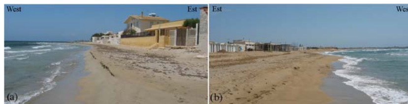
Figure 2. Anthropic pressure in the studied beach: (a) central–northern beach, where buildings are about 4–5 m from the shoreline and are reached by waves during sea storms; (b) central–southern beach, where buildings are noticeably farther from the shoreline.
