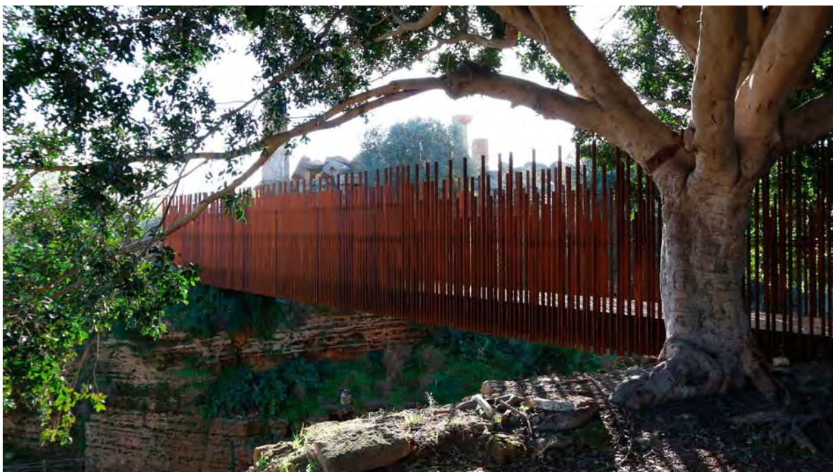
Fig. 5: Pedestrian walkway provided by Pilot Project no. 1.
