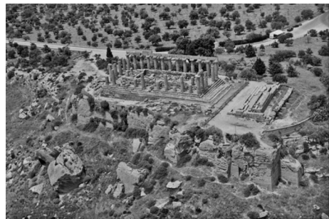
Figure 4. Aerial photo of the Temple of Hera: Note the fallen blocks and the fractured cliff face.
