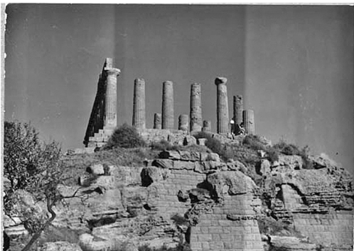
Figure 5. Old photograph showing the underlying retaining structure beneath the western cliff of the Temple.
