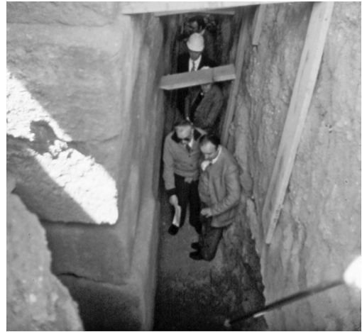
Figure 6. The Temple foundations.
