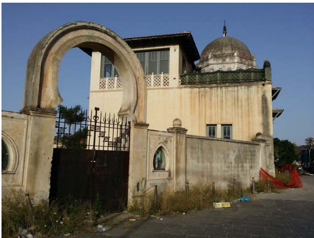
Figure 8, Stand Florio, Palermo, Sicily. The construction degrade the east facade.
