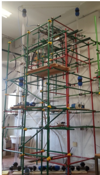
Figure 3.7 Assembling and construction of the external loop Air-Lift apparatus.
