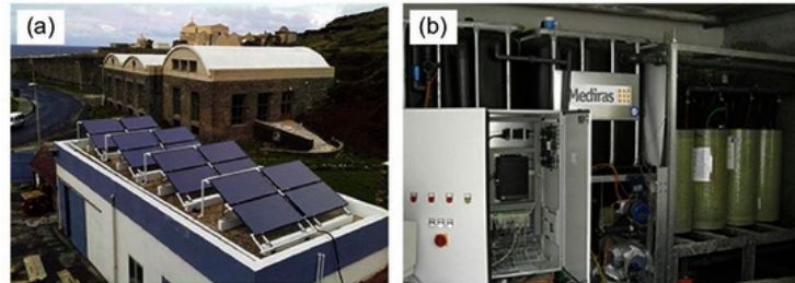
Figure 9. MEDIRAS project MD pilot plant installed in Pantelleria, (a) PV systems; (b) desalination plant pilot obtained from Viola [16], with permission Licensed under CC BY-NC 4.0 from International Journal of Heat and Technology, 2016.
