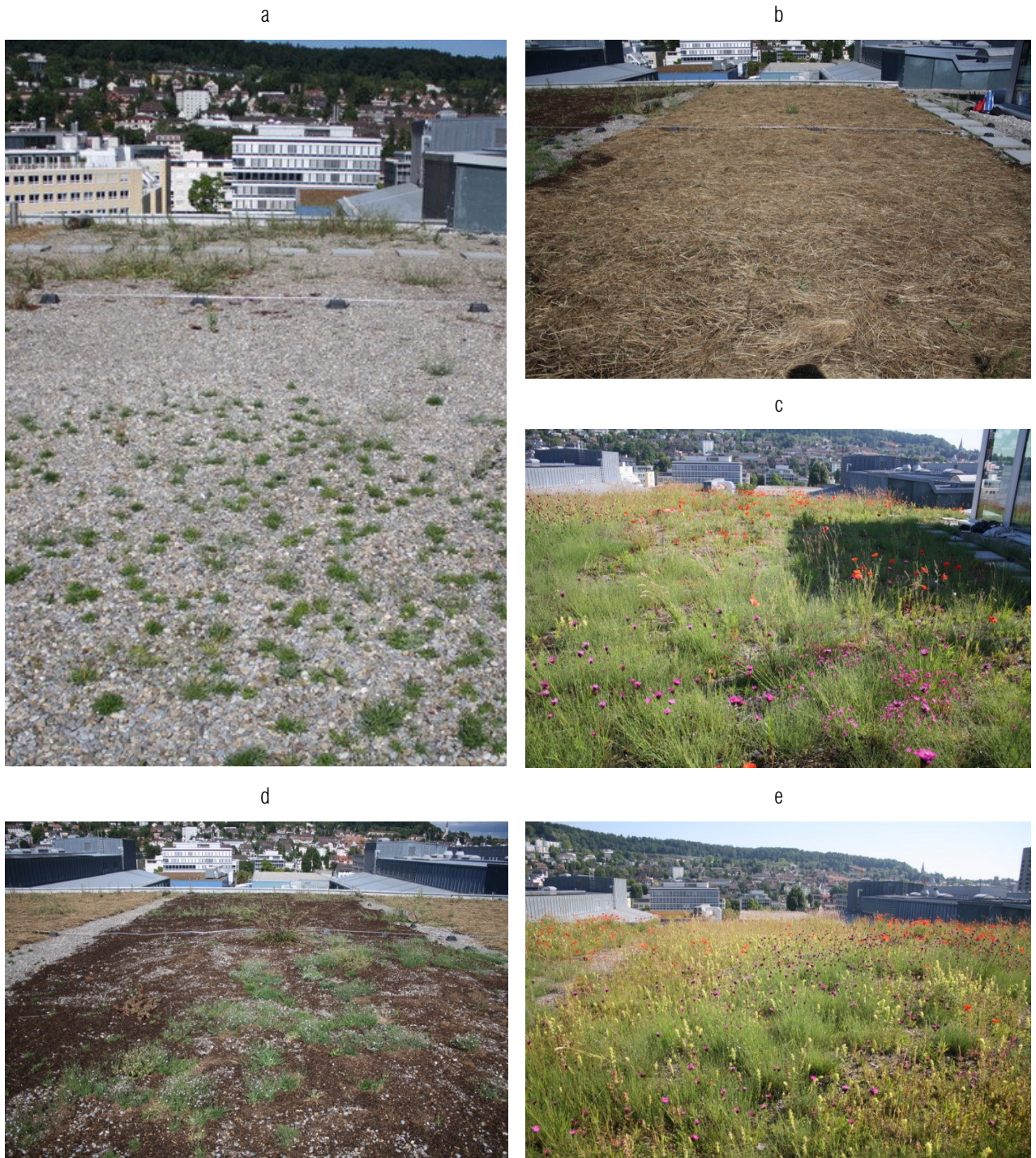
Figure 2. Hay transfer method (known also as mulching technique) applied on the green roof of Technopark in Zurich. a) roof (sandy-gravel substrate with scarce vegetation) prior to the intervention, b) laying of ca. 2 cm commercial garden substrate and fresh hay collected in September from the Zurich Lake water plant green roof in Wollishofen, c) result of the installation after a year, d) laying of ca 2 cm commercial garden substrate and sowing of seeds from threshed hay collected from July to September from the Zurich Lake water plant green roof in Wollishofen, e) result of the installation after a year
