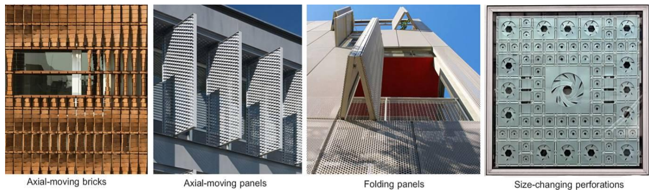
Figure 4.4: Different examples of dynamic/openable perforated envelopes, references from left to right: http://www.domusweb.it/en/news/2016/05/03/studio_admun_cloaked_in_bricks.html , https://it.pinterest.com/pin/442619469602168849/ , http://www.dezeen.com/2010/05/25/cherokee-by-pugh-scarpa/ , https://alastairgordonwalltowall.files.wordpress.com/2016/05/e4839d983ec329aa5299e38973aae77b.jpg , all accessed on (05/2016).
