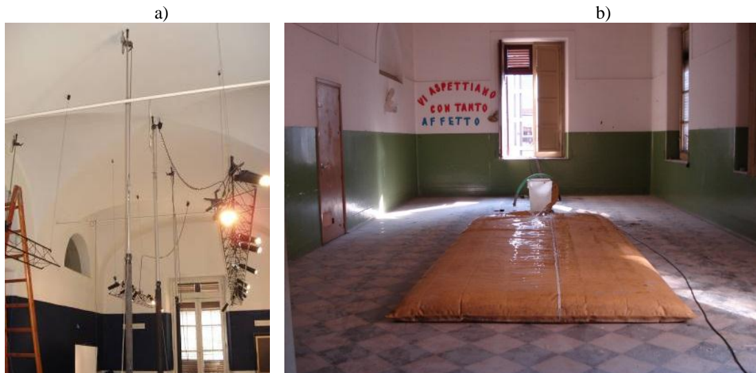
Fig. 7 Loading scheme and test set-up for loading test on Catalan vault
