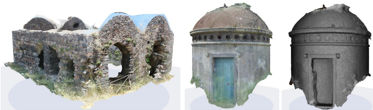
Fig. 9: 3D models of the thermal baths exterior and the second cistern both in textured and in wireframe mode.
