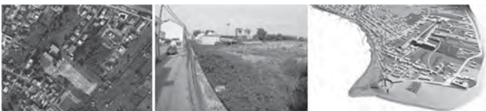
Figure 5: Messina, Torre Faro, realization of a parking.
