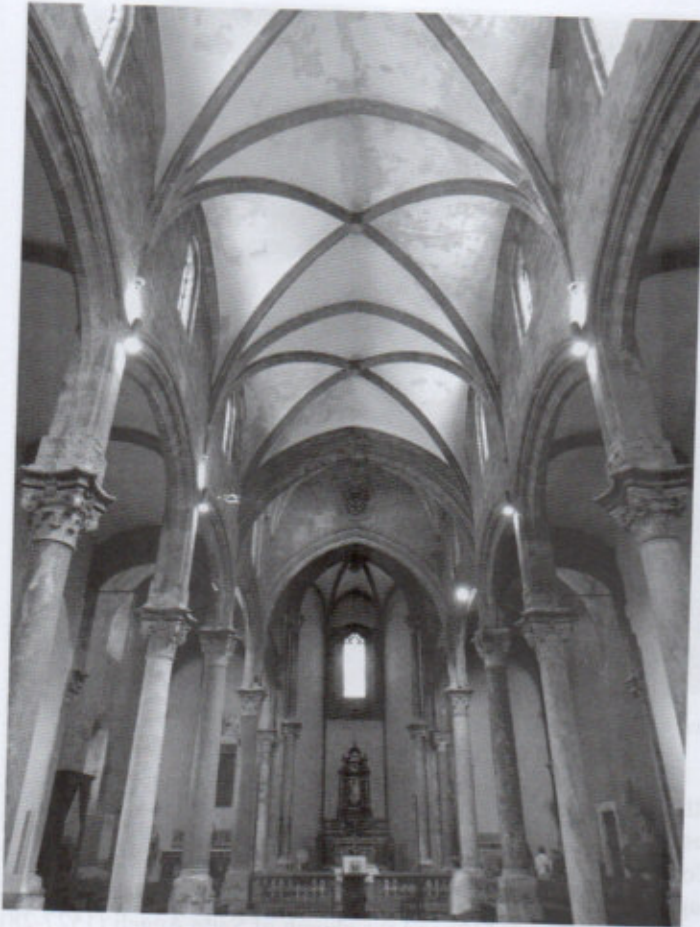
Illustration n° 3. Church of the Catena, vaults (Palermo).
