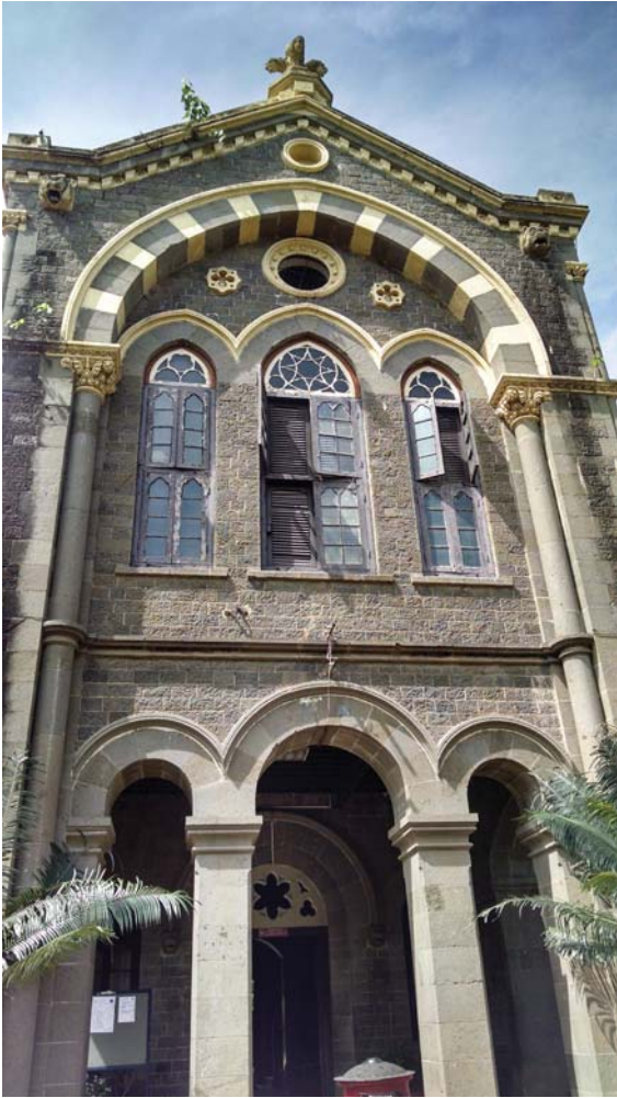
Fig. 129, Use of Polychromatic stone and window tracery work in Fergusson college photo by Lavand Vaidehi
