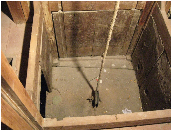
Figure 16. Path of the traction rope for the central table descent, underground from the centre of the scaffolding to the winch of Fig. 17.
