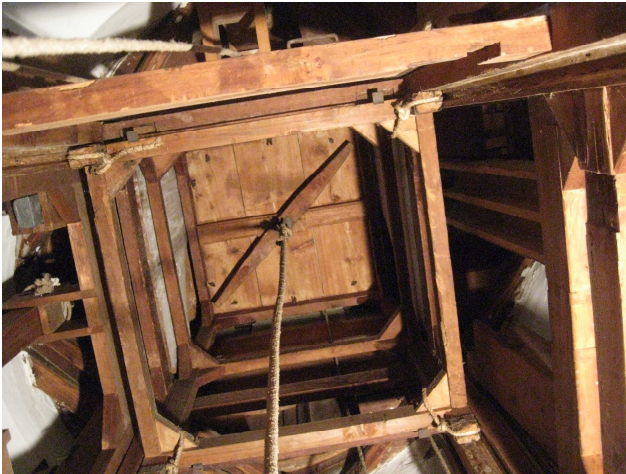
Figure 14. Sliding central frame of the table. The central rope may be drawn from below, through a couple of underground pulleys, by a monkey winch on the side of the scaffolding. Four ropes are fixed at the corners and permit to lift the frame from below by means of eight upper pulleys which return the ropes downward.
