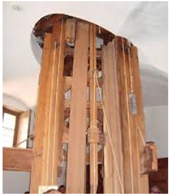
Figure 12. The lifting apparatus of the table.
