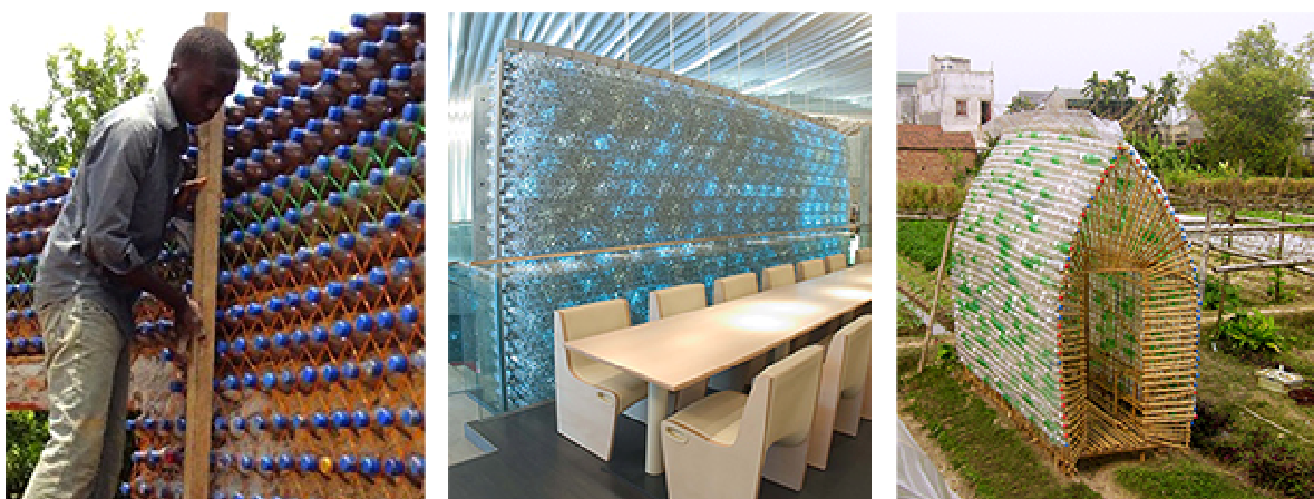
Figure 1. Three different reuses of plastic bottles in architecture: Plastic bottle house in Nigeria (a), Morimoto restaurant in New York (b), Vegetable nursery house in Vietnam (c).
