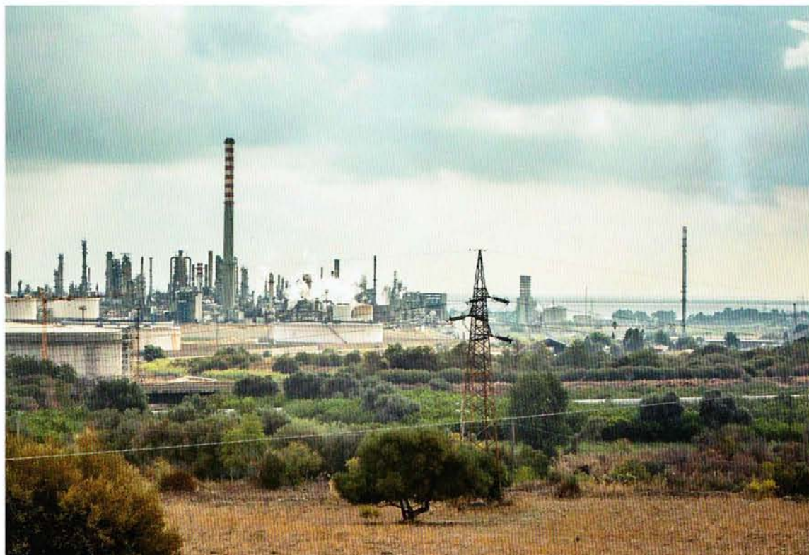
A view of the polluted industrial area surrounding the Augusta Power Station (far right).
