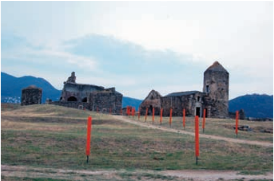
Catalonia, park of Ciutadella de Roses: view of artificial lighting equipment next to Medieval Monastery (photo by Santina Di Salvo, 2010).
