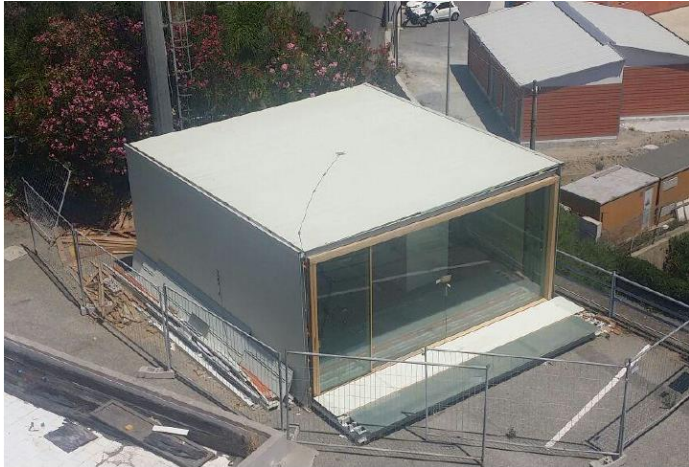
Fig. 1 Aerial view of the prefabricated module immediately after the construction stage
