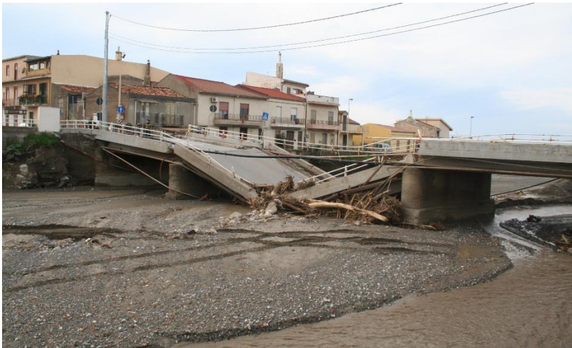
Figure 25. Photoshoot of 22 November 2011 flood event: bridge collapsed in Barcellona Pozzo di Gotto.
