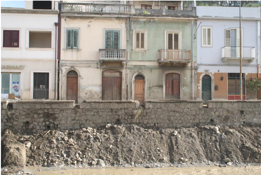
Figure 9. Example of buildings categorized as “poorly finished”.
