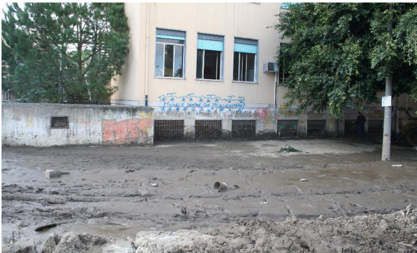
Figure 23. Photoshoot of 22 November 2011 flood event: flooded high school with basement in Barcellona Pozzo di Gotto.
