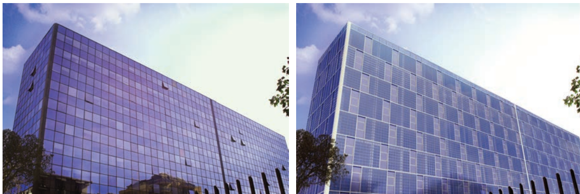
Figure 6.22 - Picture of the building at current state and rendered view of the reconfigured building envelope configuration (Tutone, 2015; Milia, 2015)
