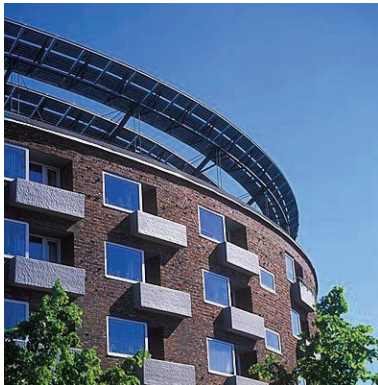
Photo 10 - Rear view of the BAPV system retrofitted on Solgården roof, Kolding
