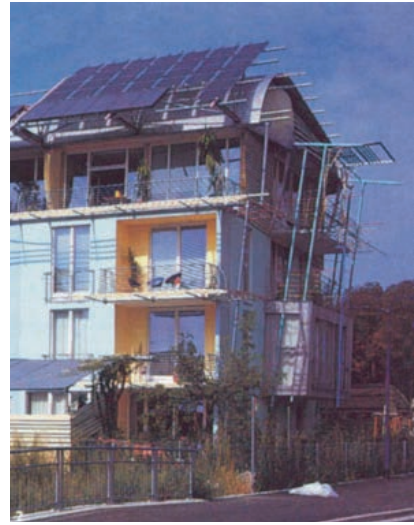
Photo 4 - Added PV system on the roof of Solar Townhouses, Freiburg-Riesefeld, T. Spiegelhalter, 1998
