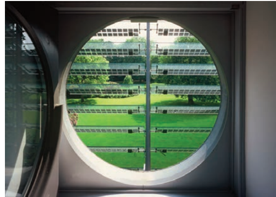
Photo 42 - View of the PV louvers installed in the field of Groenhof Castle, Flanders, Samyn and Partners, 1999
