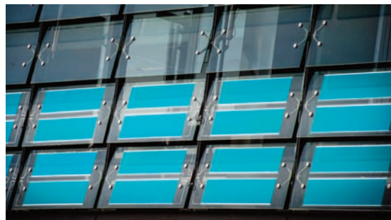
Photo 21 - Heliatek's HQ, Dresden: Heliacell laminated into glass by AGC Glass Europe, installed as sunshades
