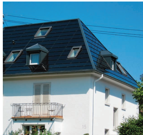
Photo 18 - Example of Cadmium Telluride photovoltaic modules integrated as roof elements
