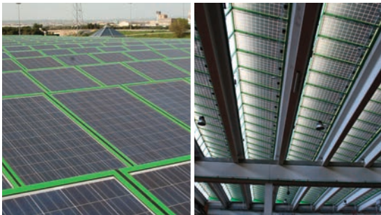
Photo 31 - Prefabricated modules for saw-tooth roof manufactured by Coversun, Cappello Group
