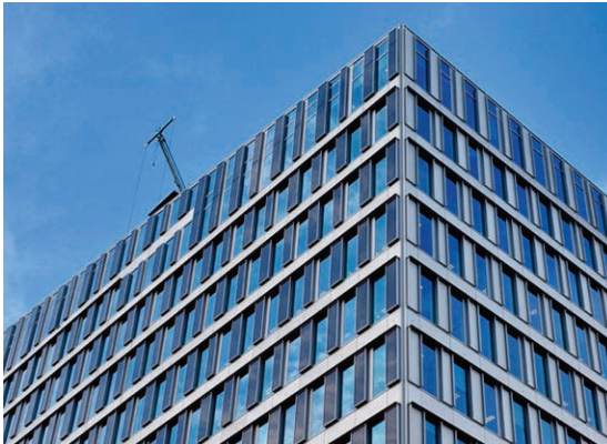
Photo 41 - View of the PV shutters at "The Edge" De-loitte Building, PLP Architects, Amsterdam, 2014
