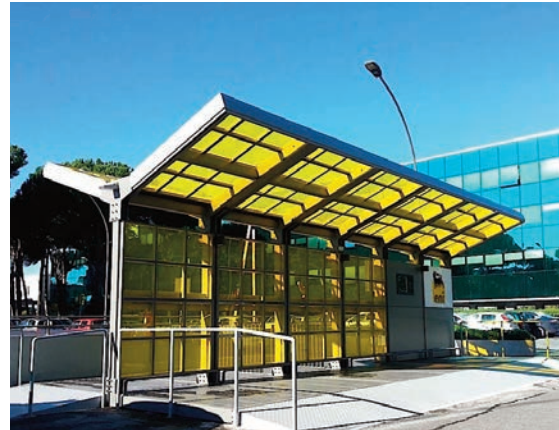
Photo 44 - Shelter for recharging electric bicycles integrated with yellow LSCs at the Division Refining & Marketing of Eni, Rome
