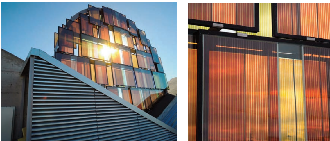
Photo 29 - The Sun at the Austrian Pavilion of Milan Expo 2015: multi-color DSC façade, manufactured by g2e and FIBAG, integrated with lighting elements for night-time illumination; (left) general view; (right) detailed view
