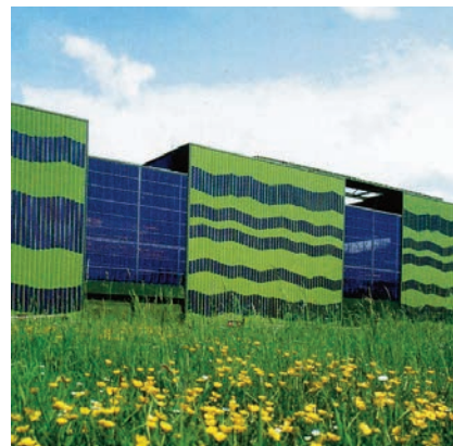
Photo 37 - ThyssenKrupp Steel Building, Duisburg, Cerny Gunia, 2002: PV-integrated blue and green façade
