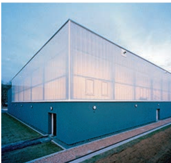
Photo 3 - Polycarbonate panels with aerogel insulation: School Gymnasium, Pbr Planungsbüro Rohling, Mainz
