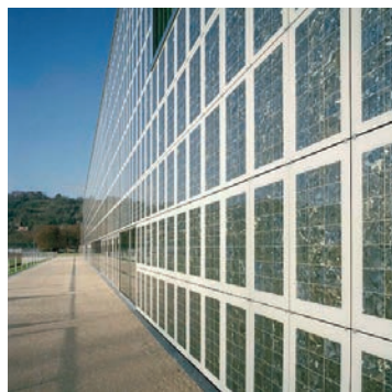
Photo 39 - Paul Horn Arena, Tübingen 2004: PV façade in green pc-Si panels (Sunways) with point supports
