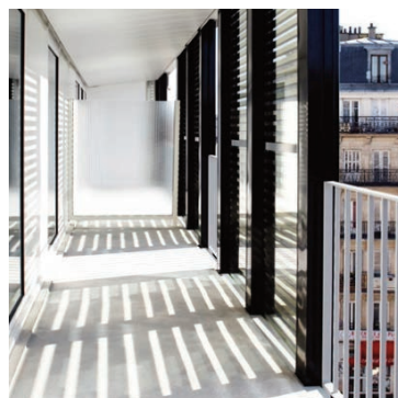
Photo 12 - Evacuated tubes as façade elements of Social housing in Rue de la Cabonnière, Philippon-Kalt, Paris, 2010
