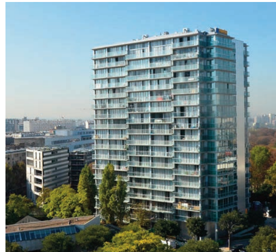
Photo 7 - Sun spaces added in the renovation of Tour Bois-le-Prêtre, Druot Lacaton and Vassal, Paris, 2012
