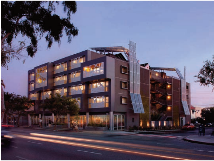
Photo 3 - Added Photovoltaic system on the façade and roof of the Sierra Bonita Affordable Housing, West Hollywood, Patrick Tighe Architecture, 2010
