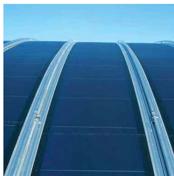
Photo 33 - Close view of Enercover installed as roof cladding
