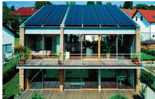
Photo 9 - PV system on the roof of a single-family house, Hegenlohe, Tina Wolfe & Michael Resch, 2003
