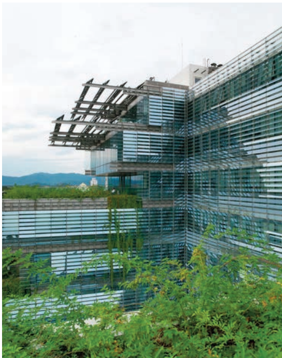
Photo 1 - SIEEB, Mario Cucinella Architects, 2006: View from the inner court of the PV panels installed as sunshading elements of building south-facing terraces
