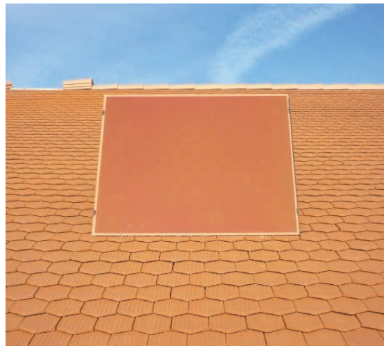
Photo 48 - Terracotta-like thin film modules for integration in heritage contexts, developed by Archinsolar (based on CSEM technology)
