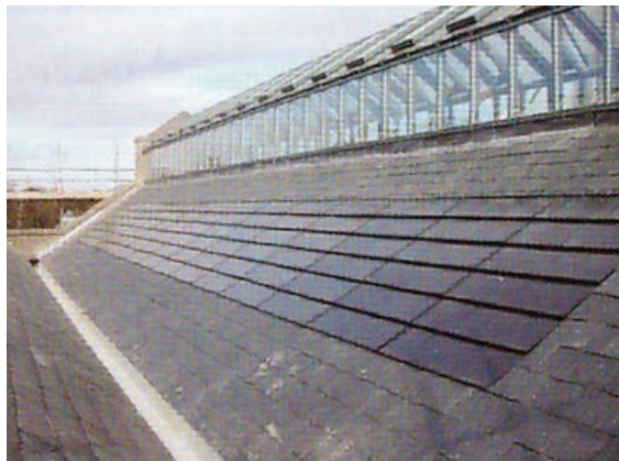
Photo 15 - PV slates integrated in the roof of Power House at Royal Gunpowder Mill, Waltham Abbey
