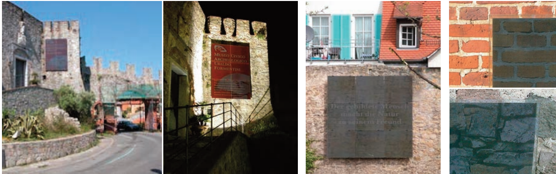
Photo 52 - PV Accept outcomes: (left) informative PV installation, S. Giorgio Castle, La Spezia; (middle) informative PV installation, Historical Centre, Marbach am Neckar; (right) semitransparent product adapted for natural stone and brick
