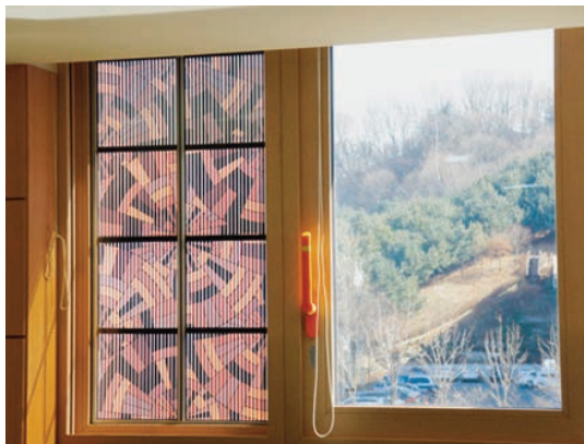
Photo 27 - DSC Solar Windows at Seoul City’s Human Resources Development Centre office complex, Seoul, 2012: view from the inside
