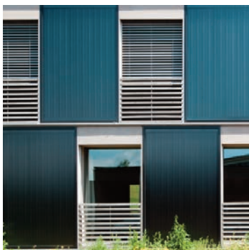
Photo 11 - Flat-plate glazed collectors integrated in the façade of Kraftwerk B, Bennau, Grab architekten, 2009
