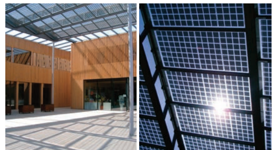
Photo 32 - Open saw-tooth roof at Ludesch Town Hall, 2006: on the right, detail of the 3-way division of panels
