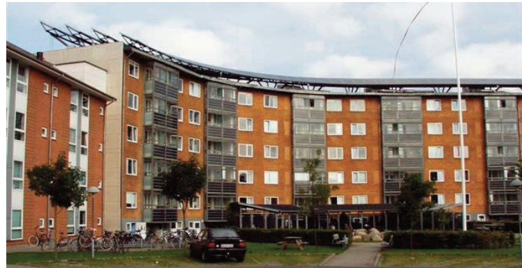
Photo 11 - View of the main façade of the Solgården, in Kolding, and of the “dominant” PV system installed on the roof
