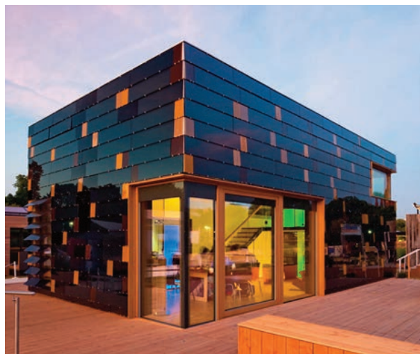
Photo 16 - Manz CIGS modules integrated as façade cladding elements in the House of the German Team (by Technical University of Darmstadt) at 2009 Solar Decathlon
