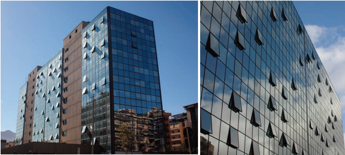
Photo 1 - Views of the building
