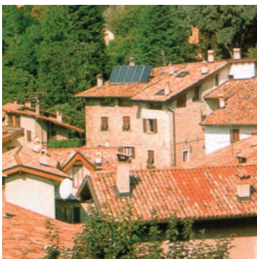
Photo 1 - PV system installed on a roof in the historical centre of Arco, Italy
