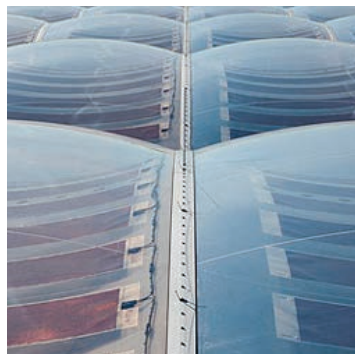
Photo 36 - AWM Carport roof, Ackermann&Partner, Munich, 2011: detail
