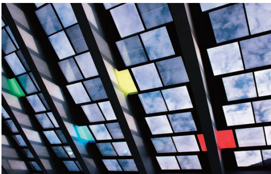
Photo 13 - Bejar Market, Salamanca, 2012: see-through a-Si modules by Onyx Solar, integrated as skylight
