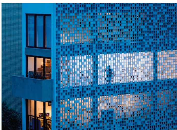
Photo 2 - Leitão_653 building, Tryptique, São Paulo, 2013: view of the "chequerboard" glass block façade
