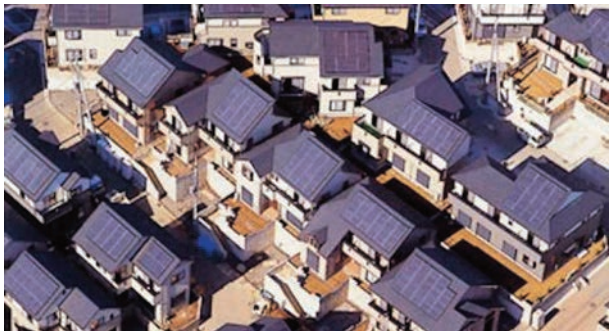
Photo 8 - PV systems on a housing district: the colour of solar panels merge with that of the roof cladding
