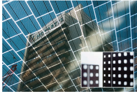
Photo 11 - Novartis Building, Frank O. Gehry, 2009 plus a detail of the solar cells used (Sunways)
