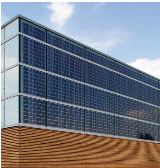
Photo 27 - Sports hall in Regensburg, Tobias Ruf, 2004. View of the south-façade integrated with PV
