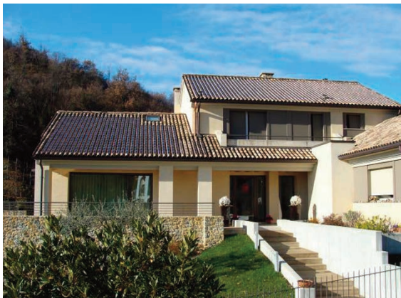
Photo 14 - Example of solar tiles (by Industrie Cotto Possagno) installed as finishing layer of a pitched roof
