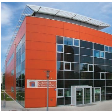
Photo 38 - Milbertshofen cultural centre, 2008: a-Si façade (VOLTARLUX®) with linear supports (Arnold Glas)
