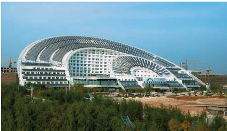
Photo 19 - Sundial Multi-purpose Building, Dezhou, China, 2009: fan-shaped roof with around 5,000 square meters of PV panel installation
