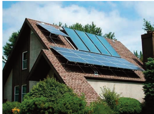
Photo 7 - Example of subjugation : PV system retrofitted on a pitched roof
