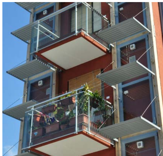
Photo 4 - Trombe-Michel wall installed in the retrofit of residential complex in Piazzale Moroni, Savona, 2003-2012
