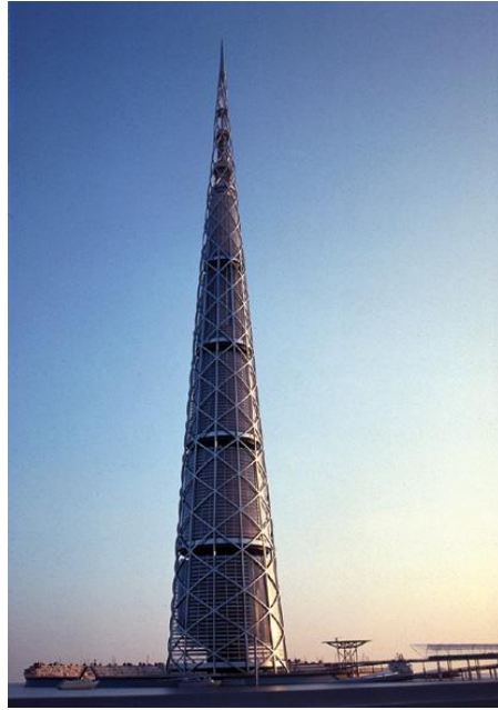
Fig. 2.13 – The Millennium Tower (Tokyo, Japan).
