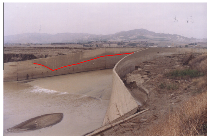
Fig. 32b. Test 6. Historical water surface profile.
