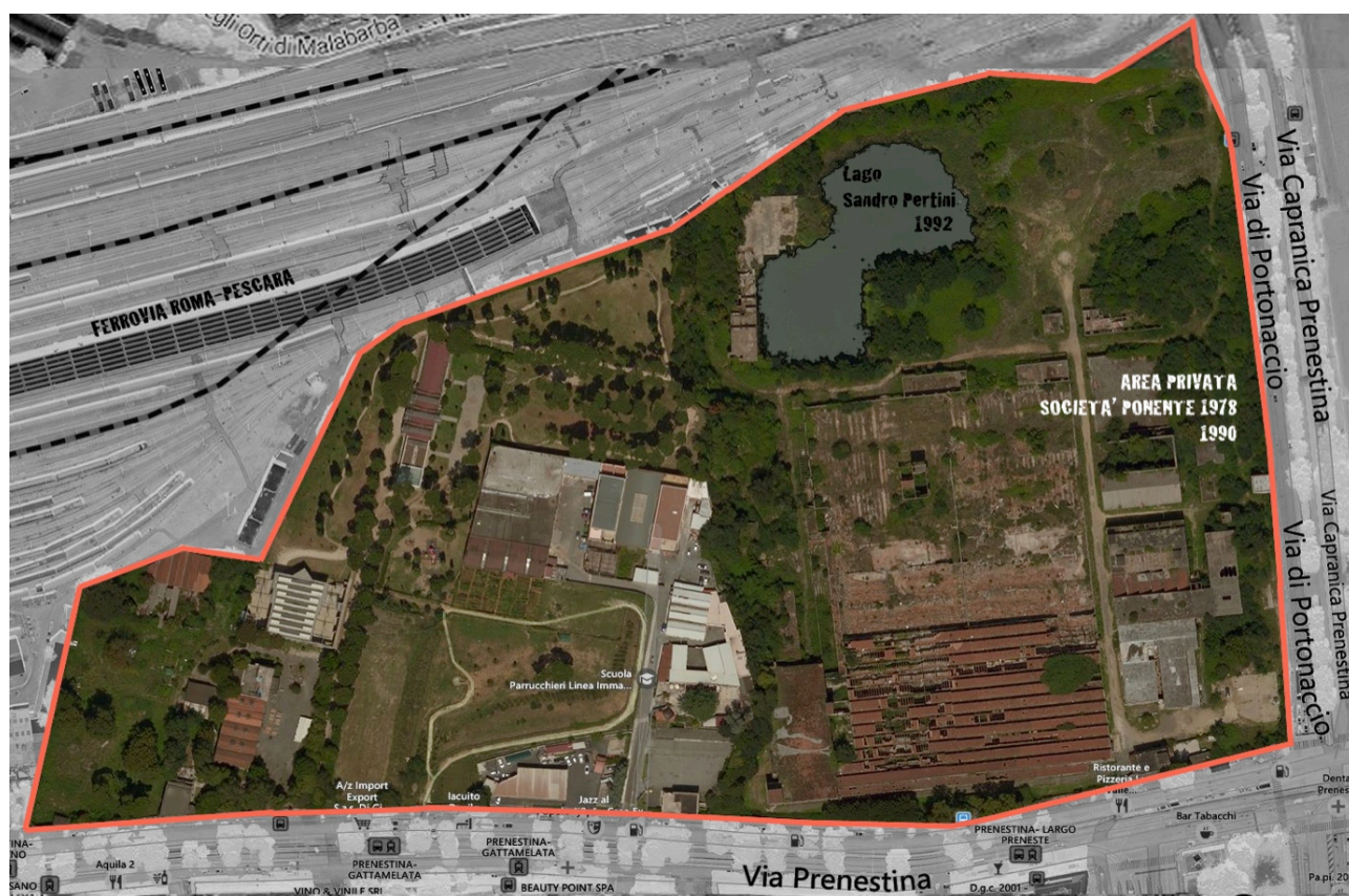
Former Snia Viscosa factory compound
