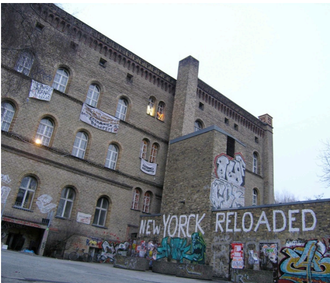
7. View of the Bethanien south-wing after the squatting action: "New Yorck Reloaded" (symbolize the re-activation of the Yorck59 project)
