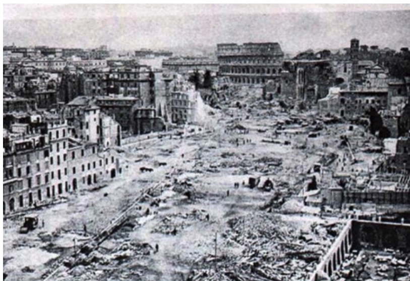
The construction of via dei Fori Imperiali and the demolition of a significant portion of Rione Monti (on the left)
