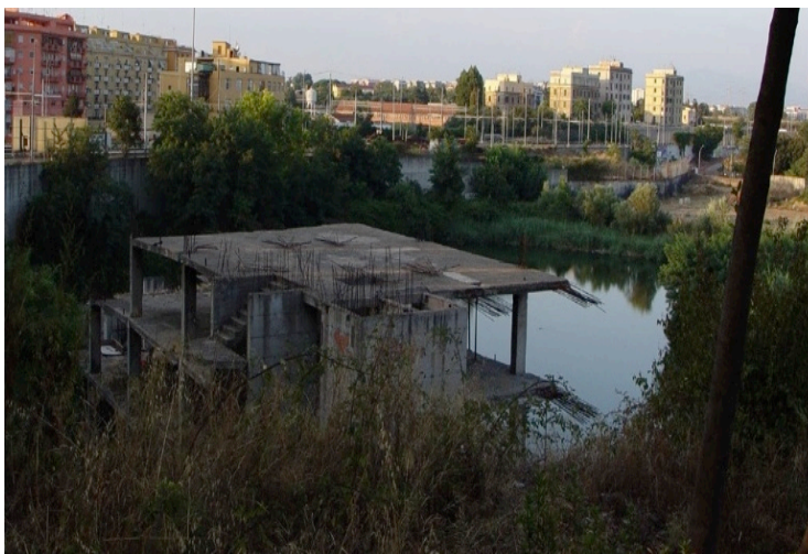
The abandoned construction site after the formation of the lake
