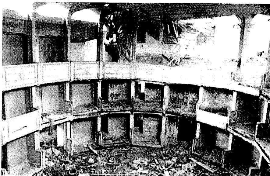
Fig. 19 Palermo, 'Teatro Garibaldi' before the interventions
