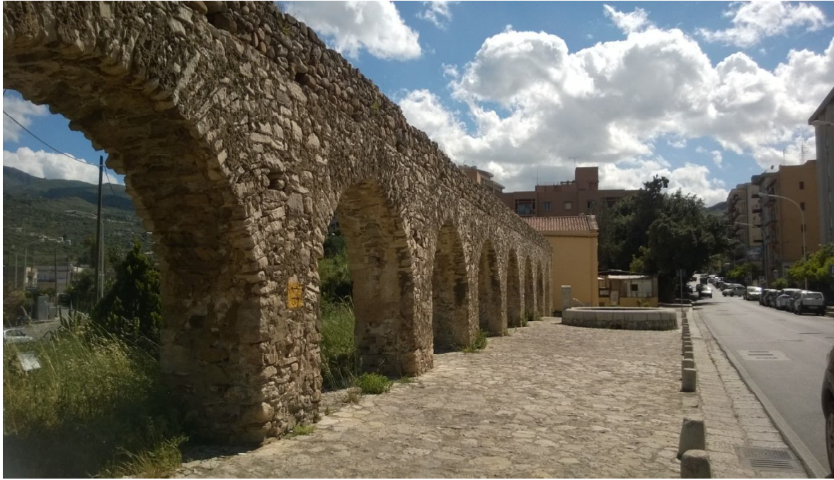
Fig. 15. Termini Imerese (IT). Aqueduct dated II-I cent. b. C., used until 1860 [photo by S. De Lisi, 2015]
