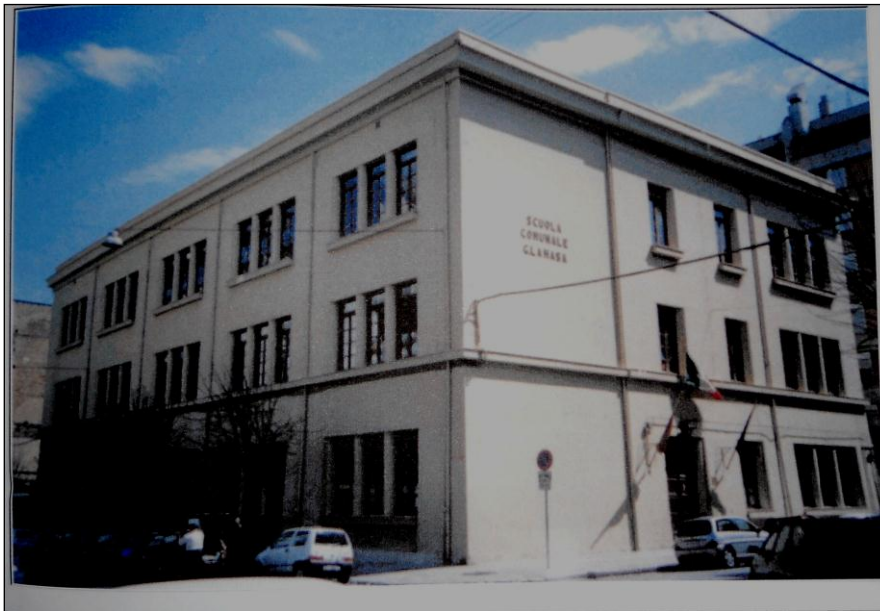
Figure 7: Photography of the school façade in 1990.
