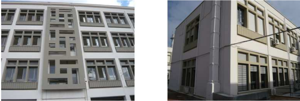
Figures 2 e 3. The brise-soleil of the body of classrooms (left) the Department of Hydraulics (right)
