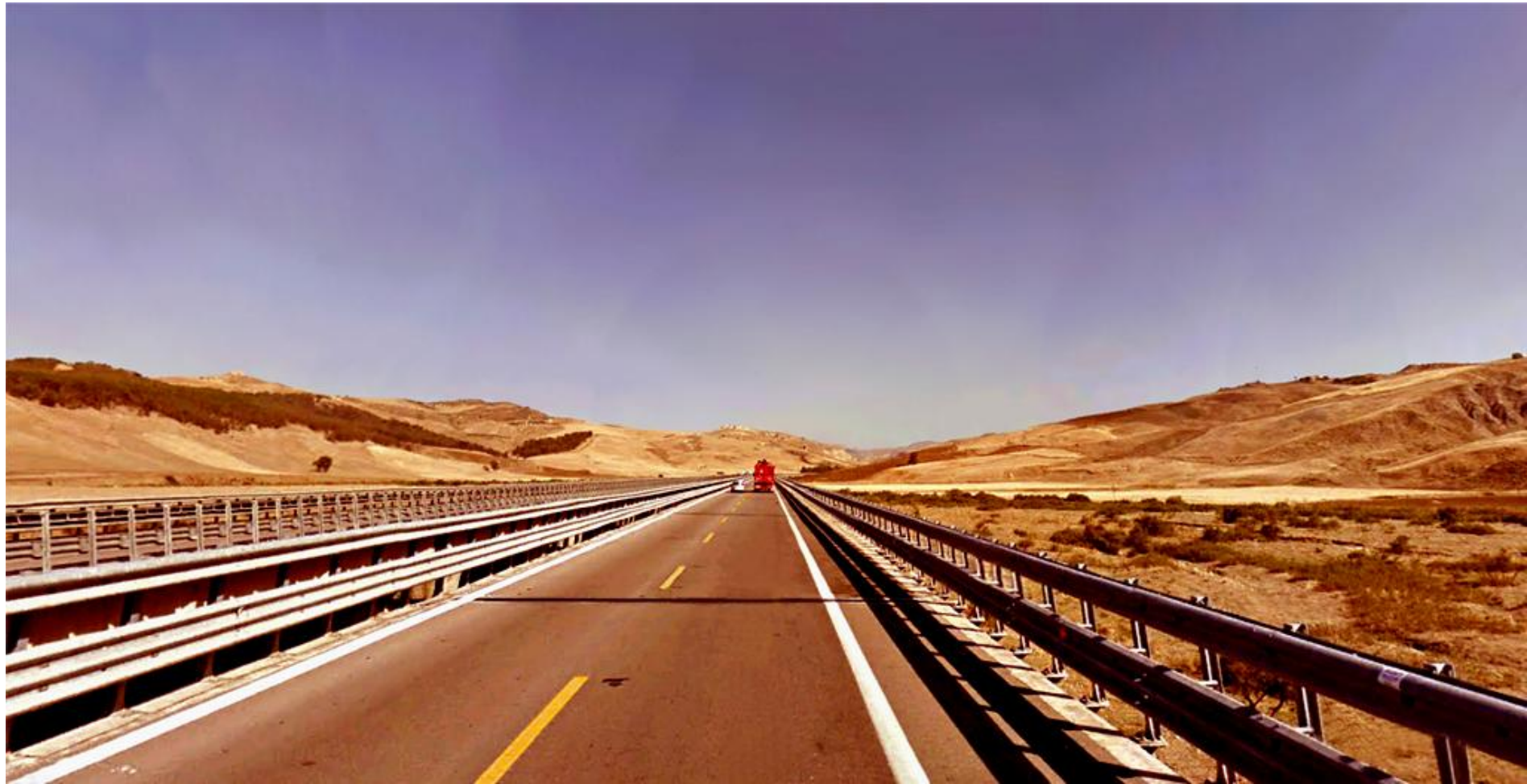
< motorway a19, viaduct crossing the dry bed of a creek
