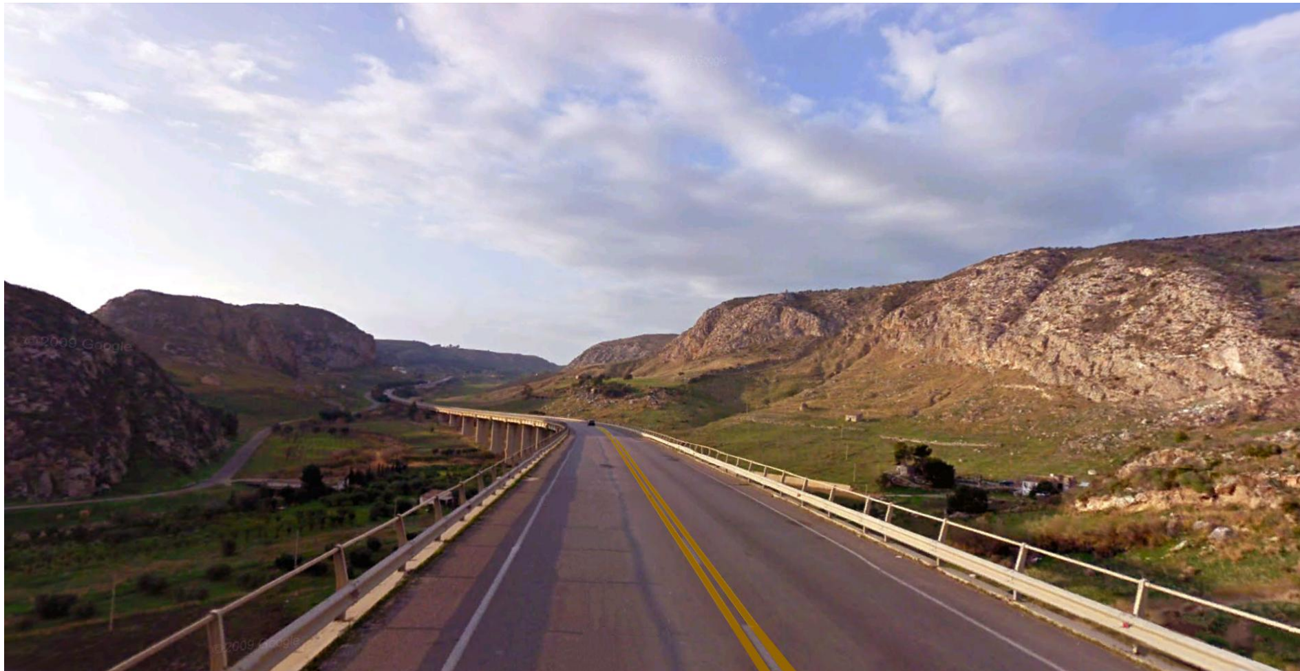
< viaduct canne, county route 75, goin' towards porto empedocle
