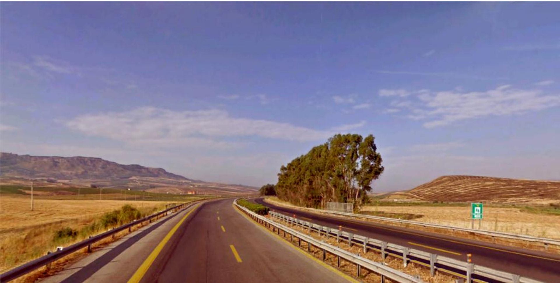
< motorway a29, approaching gallitello junction
