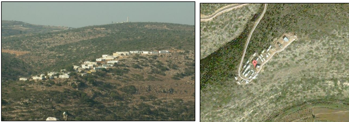
Fig. 1.10: Shilo colony was constructed on natural preserved lands. Source: http://peacenow.org.il & https://earth.google.com
