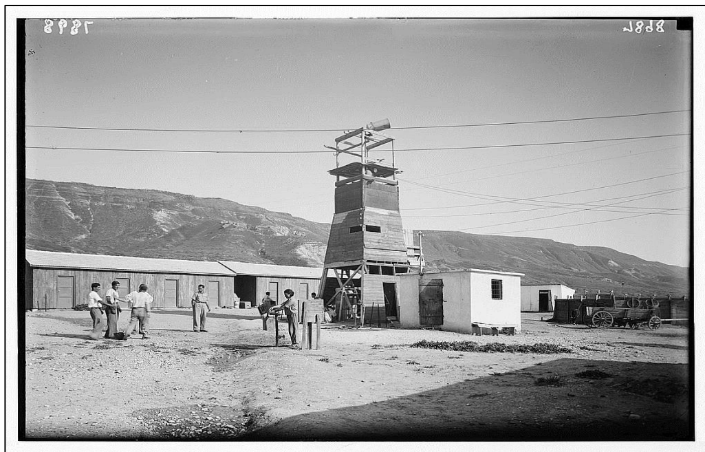
Fig. 4.7: The tower is one of main architectural element in the early Zionist and Jewish colonies.
