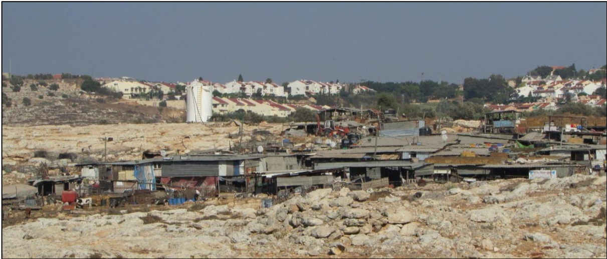
Fig. 5.11: The sharp gap of the quality of built up environment between colonizers and those who have been colonized. Source: Halawani, June, 2013
