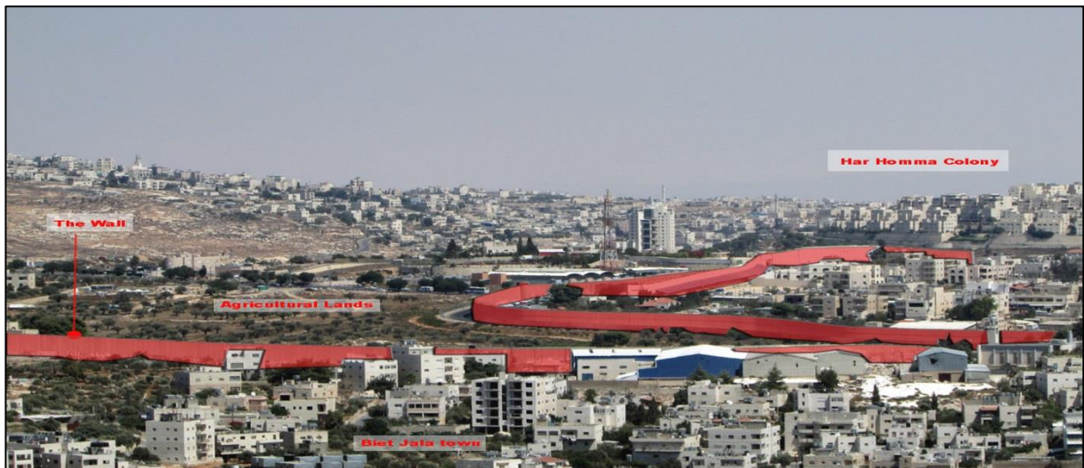
Fig. 4.17: The wall separates the agricultural lands from Beit Jala town. Source: Halawani, September, 2014
