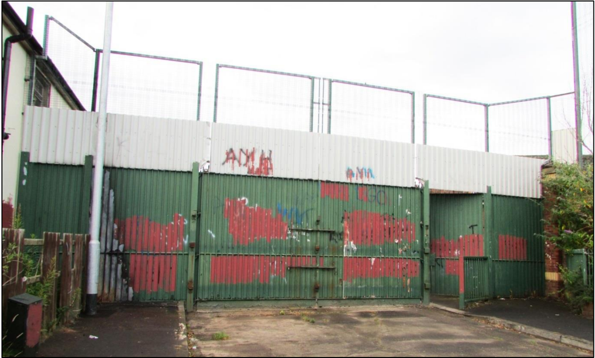
Fig. 3.1: The barrier with a gate that separates both communities (Catholic & Protestant). Source: Halawani, July, 2014
