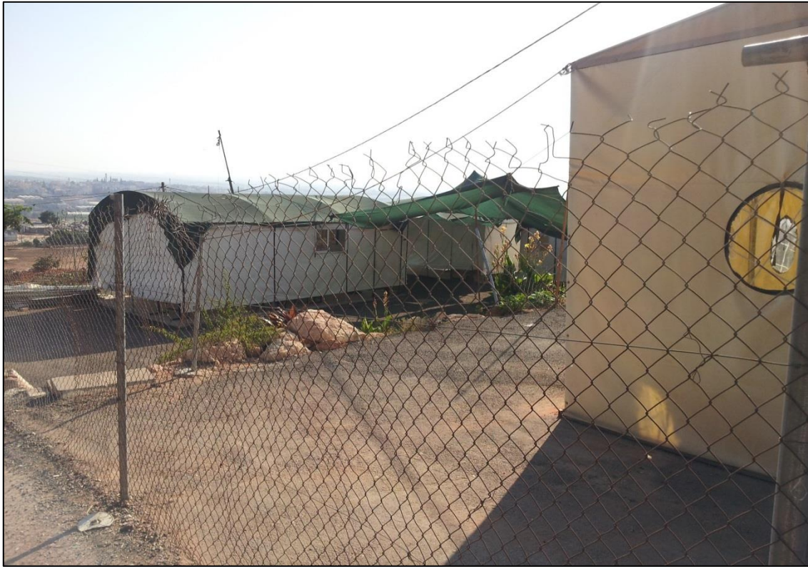
Fig. 5.31: The elementary school in A'rab ar Ramadin al Janubi. Source: Halawani, June, 2013
