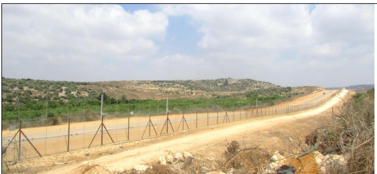
Fig. 5.22: The wall separates agricultural lands from villagers. Source: Halawani, June, 2013
