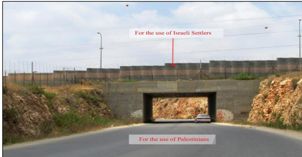
Fig. 5.32: The road is divided into two parts; the tunnel is for the use of Palestinians and the bridge is only used by Jewish Settlers. Source: Halawani, May, 2013
