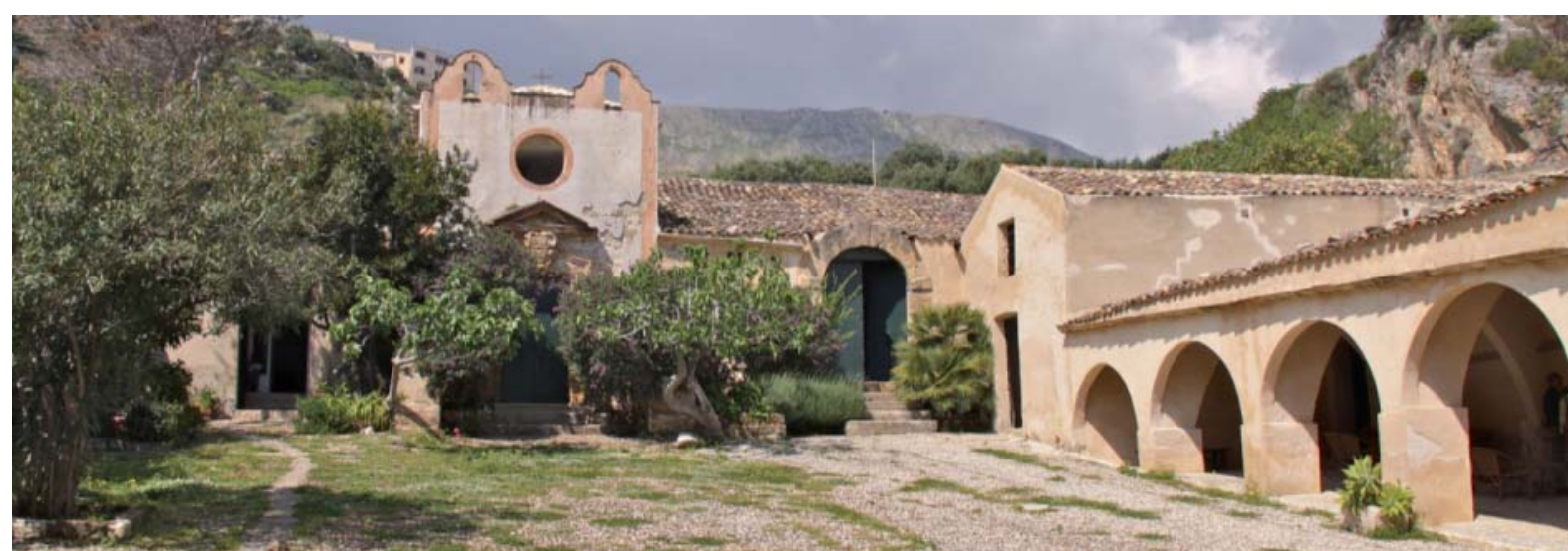
Fig.7 – Tonnara of Scopello: Warehouses (on the left side) and Marfaraggio (Archifiusis Archive); Fig.8 – Tonnara of Scopello: the court with its baroc church and on the right the so-called “appenditojo” (Archifiusis Archive)
