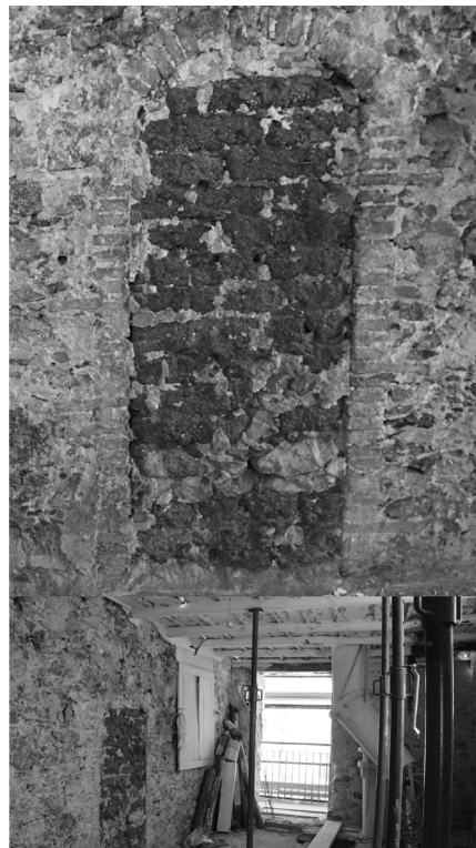
Figure 11. Empty in a stone-wall, filled-up by earth bricks, in a old building in via Vanni, Cefalù (photo by F. Vaccaro, 2013).
