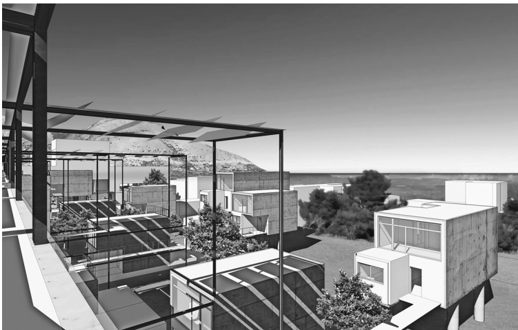
Figure 6. Solar panels shade terraces and courtyards
