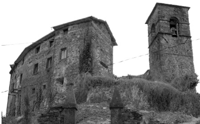
Figure 4. Picture of the encastellation complex that dominates the ridge, owned by the Bertacchi family. It is important to note the complete absence of openings in the lower part of the wall, obviously an evidence of the defensive function of the building, that is accessible only from the protected inner area of the ancient village. On the right stands out the tower bell of the destroyed church.
