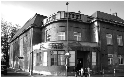
Figure 2. View of the Sokół in Sieniawa from the south-east before revalorisation, photo D. Ku nierz-Krupa, 10.2008.
