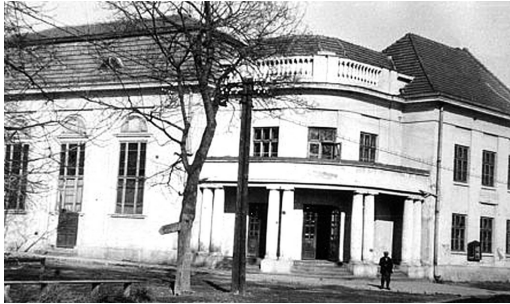
Figure 1. View of the Sokół in Sieniawa from the south in the first half of the 20th century, [in:] Archive UMiG Sieniawa, s.v.
