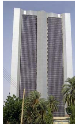
Fig. 10.22 Telecom Tower in Istanbul (Turkey) where photovoltaic modules in laminated safety glass were installed on the façade by Ertex Solar.
