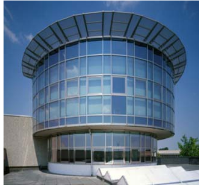
Fig. 9.15 a-b Left: Pilkington Activ™ glass had been used in the MSV Arena Soccer Stadium, Duisburg, Germany. Right: Fergamma Offices, Mantova (Italy) – 2005, where SGG Bioclean™ glass produced by Saint Gobain had been used.
