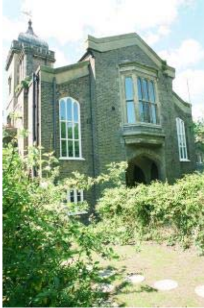
Fig. 9.18 a-b In both these buildings Pilkington Active™ glass was used. Left: the Chapel, Penge (UK). Right : Hôtel de Région, Lille (France).
