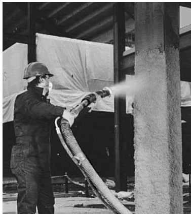
Fig. 9.37 Spray gypsum based plaster fireproofing.
