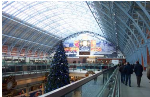
Fig. 9.16 a-b SGG Bioclean™ glass produced by Saint Gobain had been used in the arcades of S. Pancras Railway Station, London, UK (2007).
