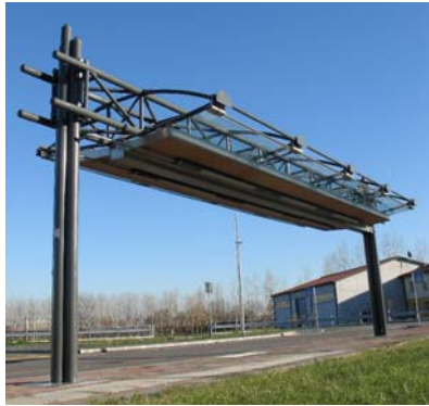
Fig. 9.19 a-b Overground shelter in Veneto (Italy) where Pilkington Activ™ glass was used.
