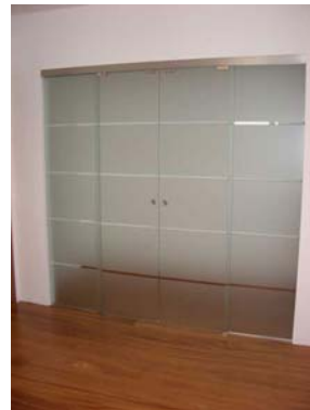
Fig. 5.8 a-b Left: steel without and with an anti-fingerprint coating. Right: a sandblasted glass door.
