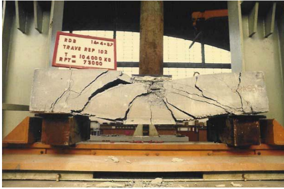
Figure 2.11. Shear failure of HSTCB.
