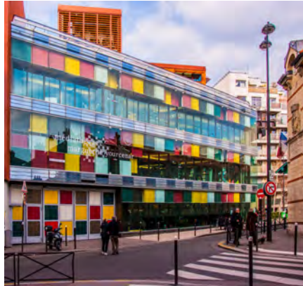
[fig. 1] Paris (France), Médiathèque Marguerite Yourcenar. View from Corbon Street. Babel Architecture. Photo by Luigi Failla.
