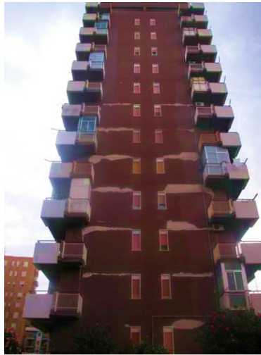
Fig. 1.6. Positive contribution of infills to earthquake resistance of a RC framed structure.
