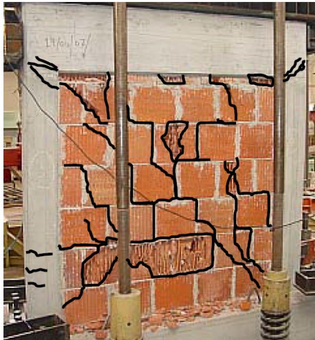
Fig. 2.28. Specimen cracking patterns at the end of test.
