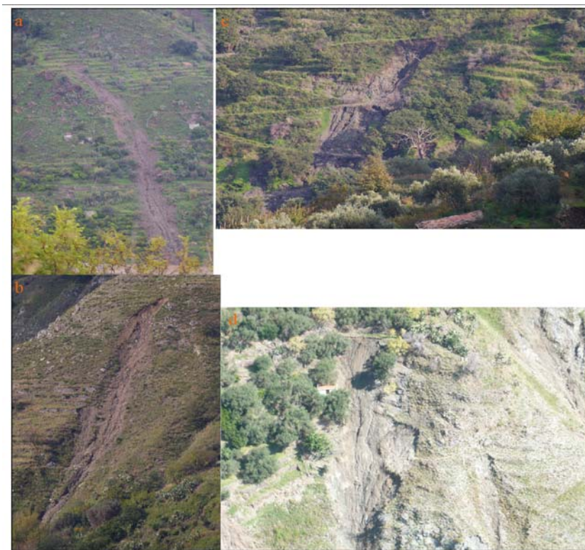
Fig. 2.20 – Examples of flows triggered by rapid flow with arched crown (a, b) or straight (c, d)
