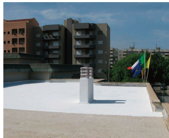
Photo 9 - Experimental cool roof made of eco-friendly white organic water paint in Trapani, Sicily
