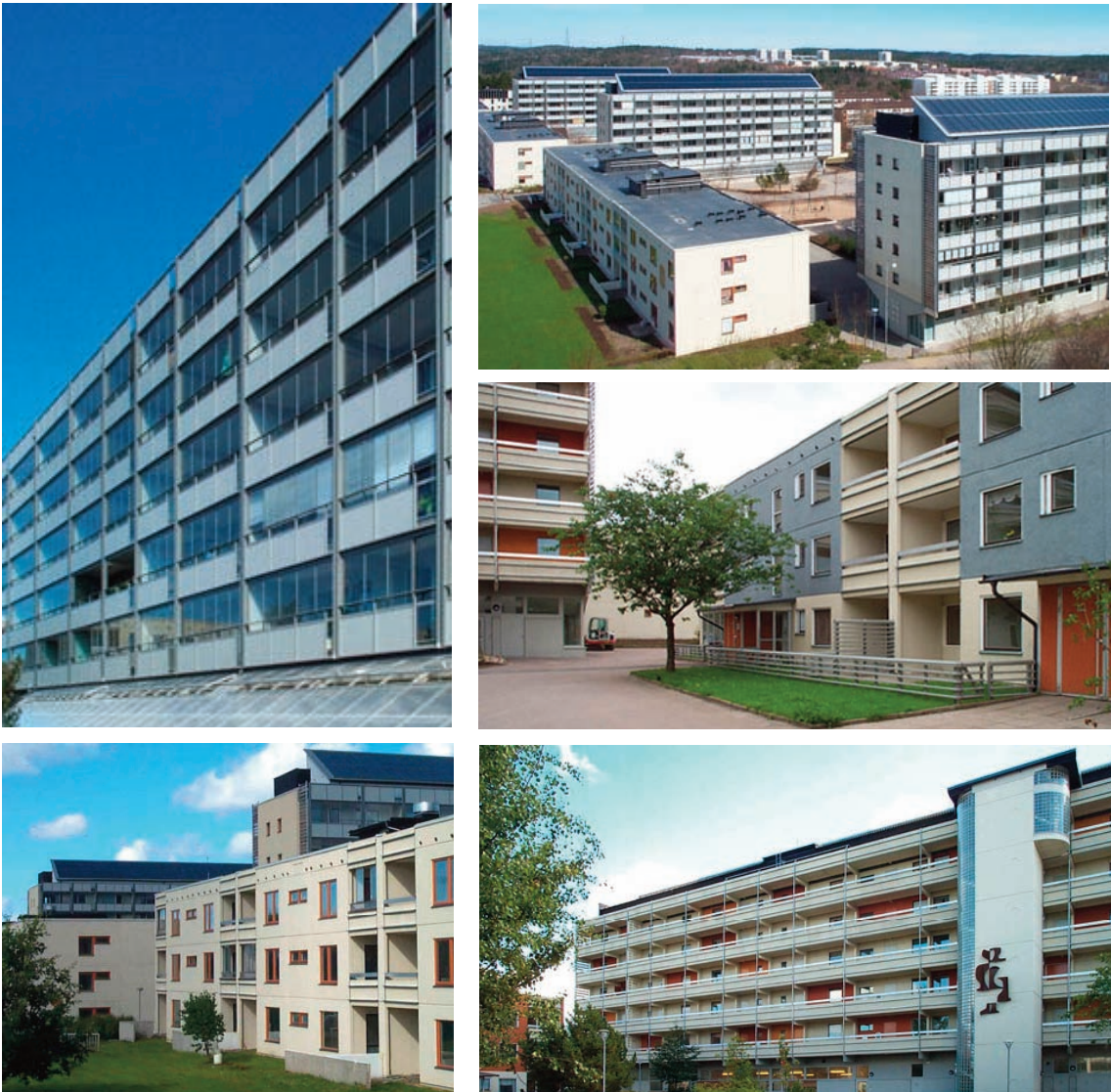
Photo 48, 49, 50, 51 and 52 - Views of the complex after retrofitting
