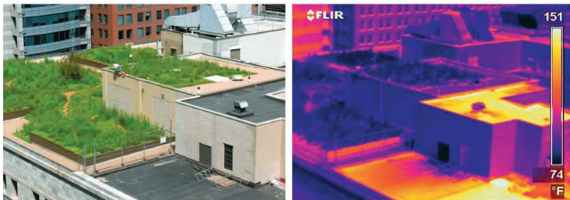
Photo 2 - Temperature differences between a green and conventional roof in Chicago
