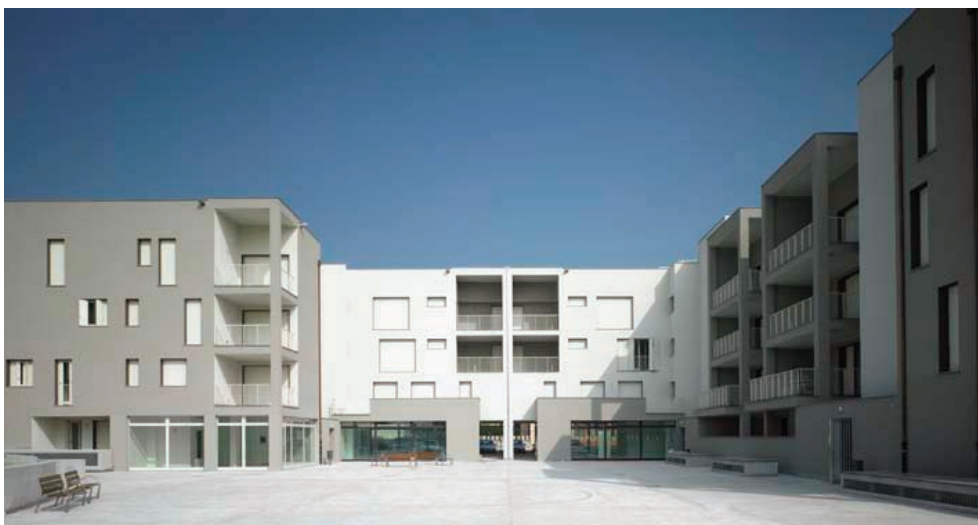
Fig. 4 - Casa Crema+, one of the project currently undergoing supported by FHS
