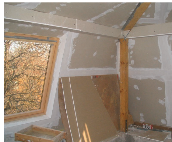
Photo 15 - Thermal insulation of the attic during retrofitting
