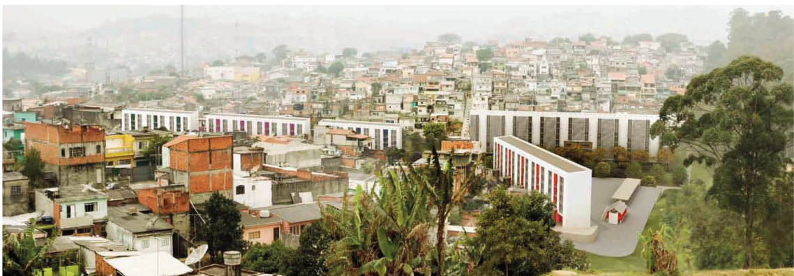
Fig. 9 - Photomontage of the new buildings in the community of Bamburral (by courtesy of Brasil Arquitetura)
