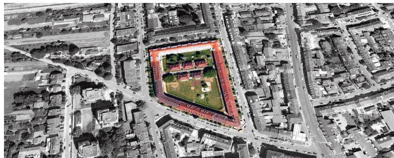
Fig. 17 - Aerial view of the housing complex
