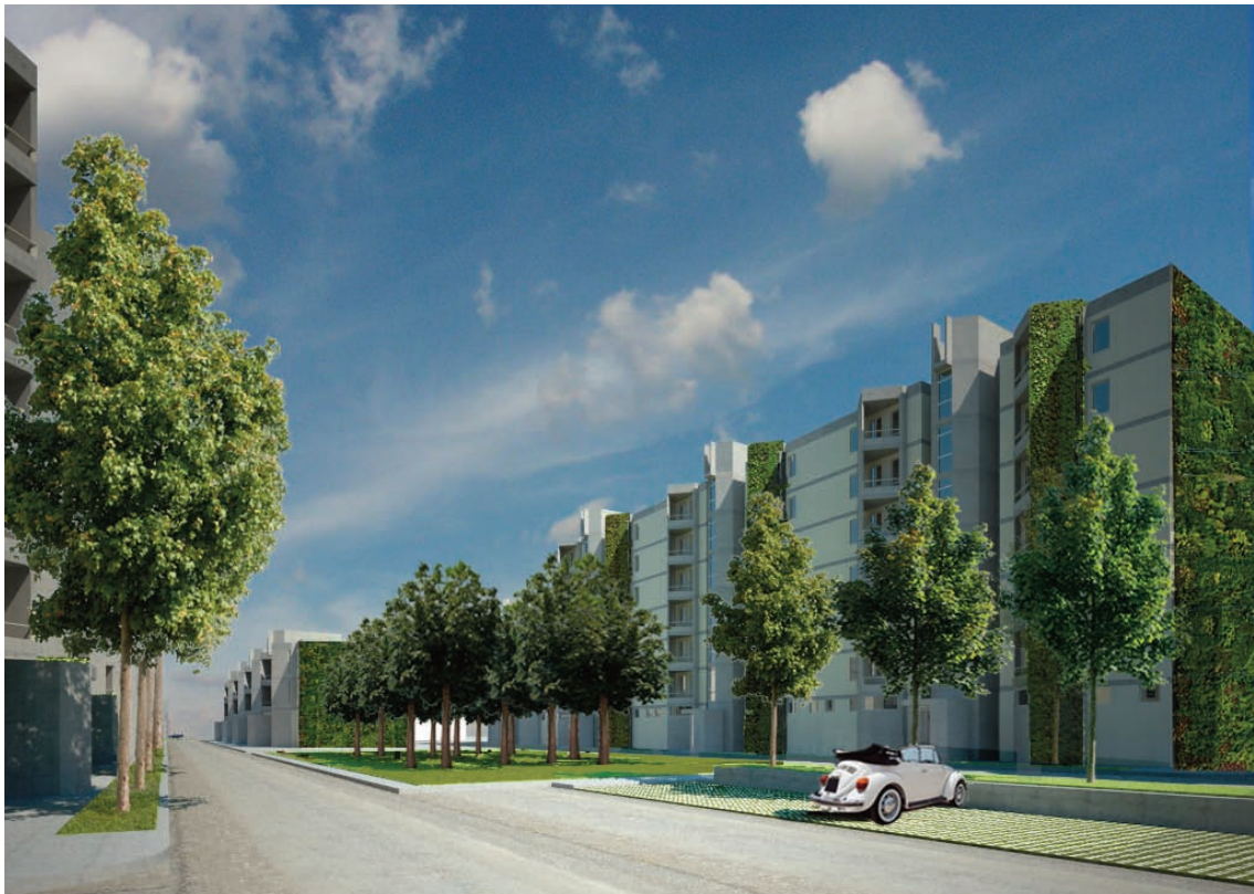
Fig. 2 - Rendered image of the Medaglie d'Oro complex after retrofitting: view of the common area
