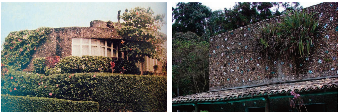
Photo 13 and 14 - The Chame-Chame house in Bahia (left) and the Cirell House (right) by Lina Bò Bardi
