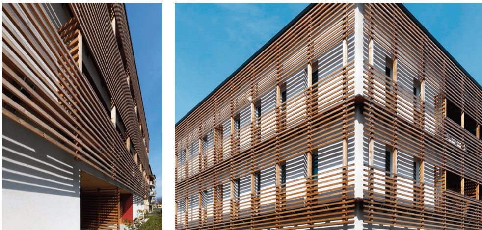
Photo 1, 2 and 3 - The collective eco-friendly building in Motta di Livenza (Treviso), designed by the architectural firm Matteo Thun & Partners
