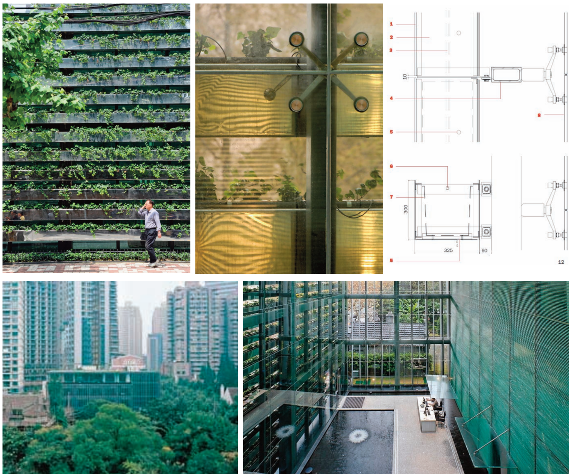
Photo 29, 30, 31, 32 - Clockwise from top left: façade with green louvers; a detail of the façade structure; an internal view and an overall view of the building. On top right: Fig. 14 - Constructive detail of the green façade
