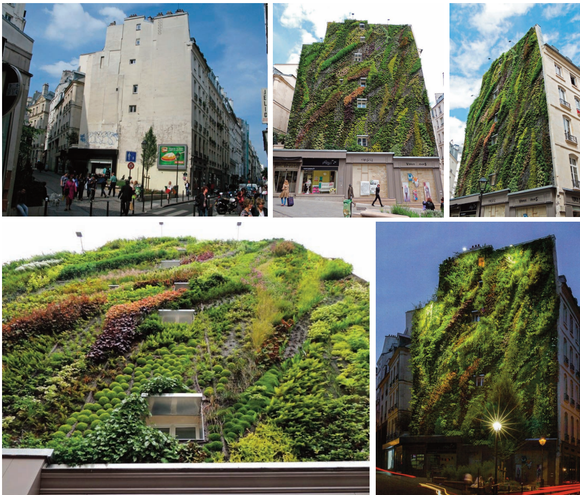
Photo 33, 34, 35, 36 and 37 - Clockwise from top left: The façade before the intervention; views of the façade after the installation of the living wall (others)
