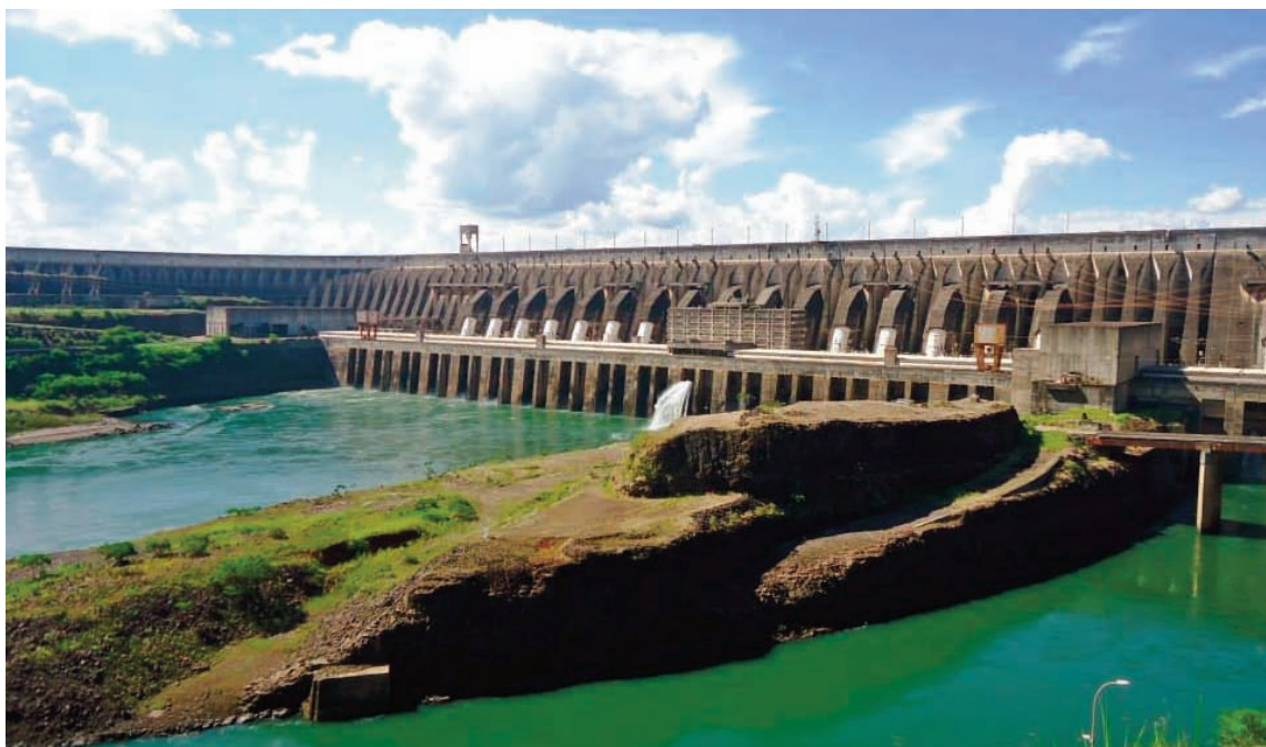
Photo 6 - Hydroelectric power plant in Foz do Iguaçu
