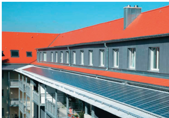
Photo 45, 46 and 47 - Insulation applied on an apartment ceiling (top left), photovoltaics panels installed at the top of the balconies (bottom left) and the new balconies with independent structure (right)
