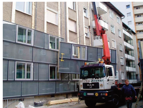
Photo 9 and 10 - Holes for the ventilation of the new façades (left) and the installation of the GAP-solar panels (right)
