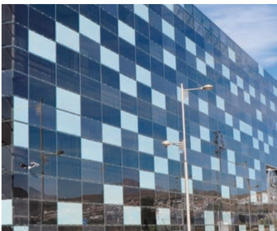
Photo 8 - Ventilated façade made of glazed, photovoltaic and opaque elements in the GENyO building of Granada
