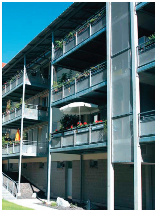
Photo 45, 46 and 47 - Insulation applied on an apartment ceiling (top left), photovoltaics panels installed at the top of the balconies (bottom left) and the new balconies with independent structure (right)
