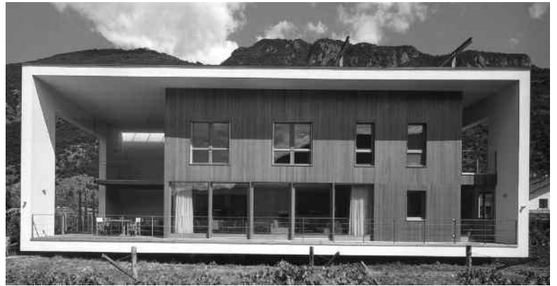
Casa Mumelter, Arch. Werner Tsholl, Gries, Bolzano 2000.
