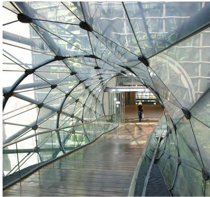
Arndale Bridge over Corporation Street, Manchester, England. (iperboloide iperbolico)
