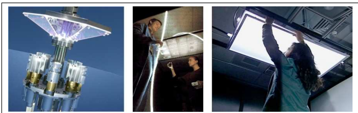
Collector and diffuser of Hybrid Lighting System.
