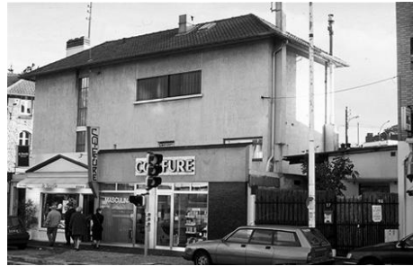
Fig. 1. Flat roofs and terraces are critical architectural choices from the hanging Babylon gardens. The pictures show the Le Corbusier villa Vaucresson, dated 1922 and its later “refurbished” version, after probable long series of water infiltrations and maintenance works through flat roof. At that time, waterproofing technology was still based on the application of thick asphalt layers, not easily turned up on walls and parapets, or on built-up bituminous roofing membranes (many fiber layers plus hot melted asphalt). Both systems were fragile at temperatures below 10°C, just few months after its application, and suffered any cracking or movement of the substrate (images from: http://www.pushpullbar.com/forums/ )
