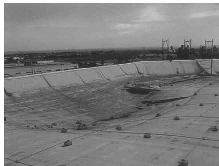
Fig. 1 Last settling of roofing
