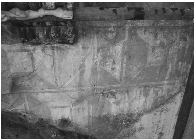
fig. 2 Degradations. Particular of the scratch ashlars below the balcony of the second floor
